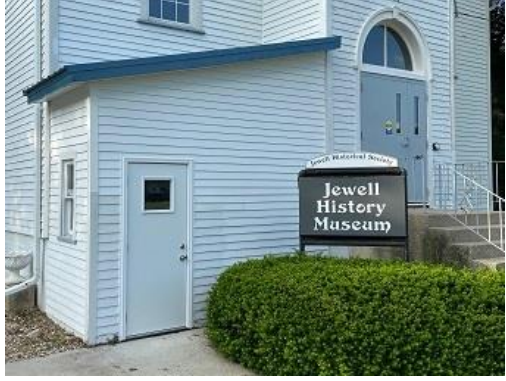
Restored Southwest Entrance
