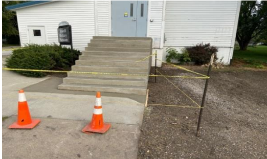
Newly-Poured Front Stairs
